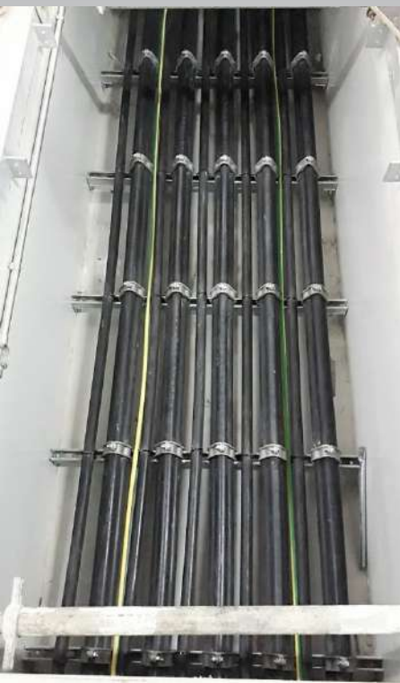
LV cable laying in trench
