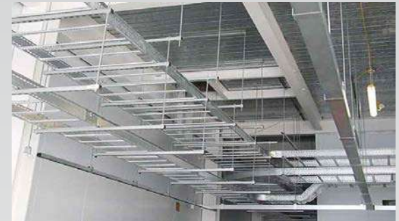
Installation of all type of containment
